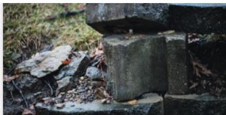
Parsonage Stonework Project
