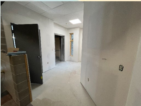
The new main level elevator lobby.
